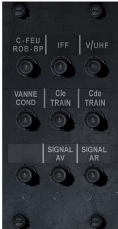
Figure 3 Circuit breaker panel
